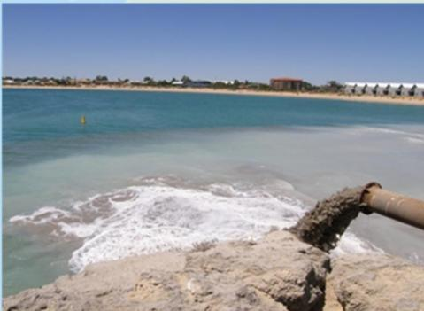
This can result in an imbalance in sediment distribution along the adjacent shorelines, leading to unnatural patterns of erosion and accretion. Sand bypassing simulates the natural longshore transport by redistributing sand from areas of accumulation to eroded sections of the coastline. This beach renourishment can be vital in preventing excessive beach erosion and preventing undermining of adjacent coastal infrastructure. Sand bypassing is
